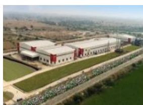
Mayur's newly commissioned PU plant in Morena, MP
